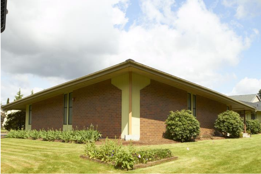
Original building on site, Grace Chapel
